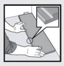
**3.** At the end of the first row, place a 1/4" spacer against the wall and measure the remaining space to determine the length of the last plank needed. Cut the last plank to the correct length, ensuring that it is at least twice the width of the plank for optimal installation.
